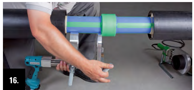
16. Open the clamping jaws of the welding jig as far that the welding jig can be removed sidewise or downward from the connection.
