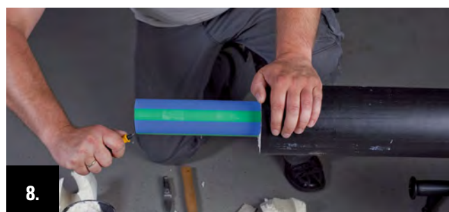
8. Clean the skinned medium pipe and deburr the pipe ends inside and outside.
