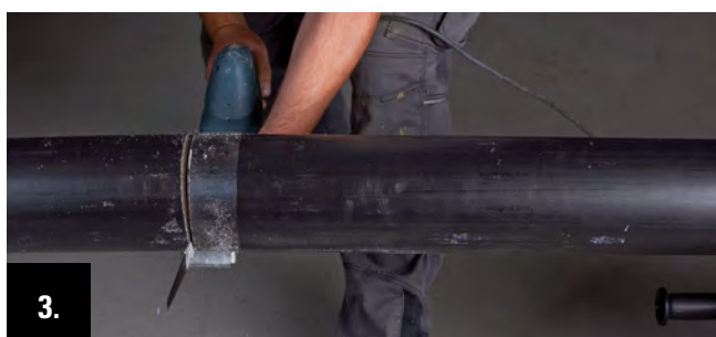
3. Cut the pipe with a customary handsaw with a saw blade for plastic along the cutting line.
