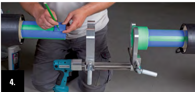
4. The welding depth and the clamping distance are marked by the aquatherm clamping template (blue) in one work.
