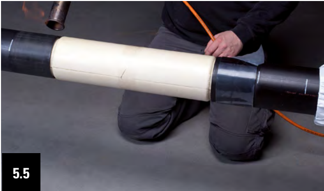
5.5 Repeat the described work process of step 5.1 to 5.4 at the other end of the casing pipe.
