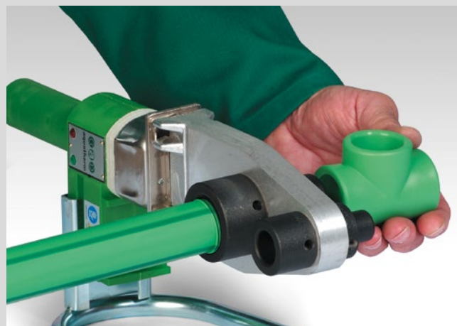
Heating-up of pipe and fitting
