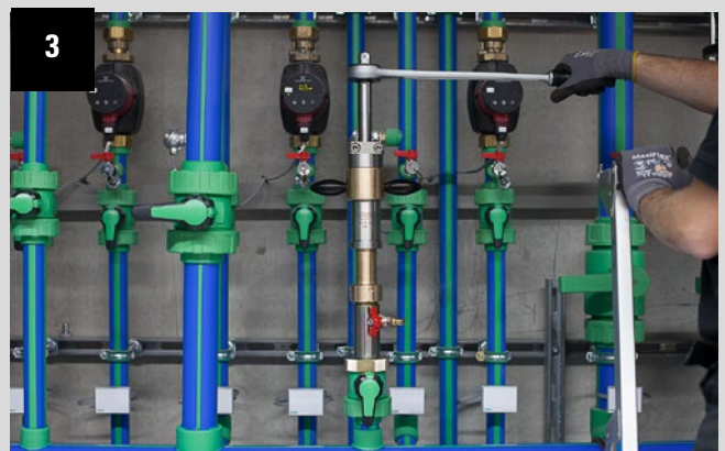
3. Start of the drilling process
