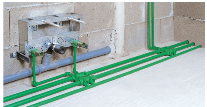
Floor distribution with distribution blocks
