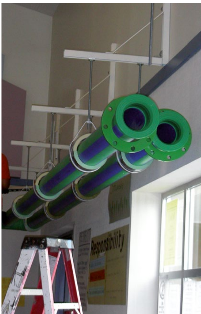
Park Orchard Elementary School, Kent (WA), USA
