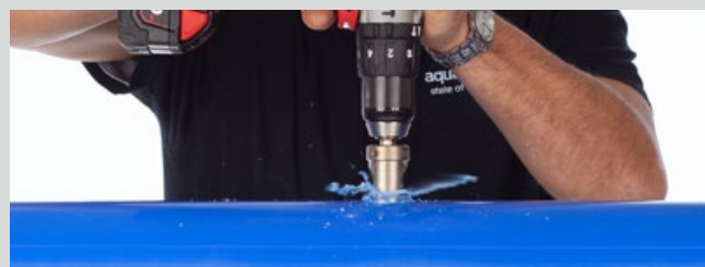
Drilling through the pipe wall
