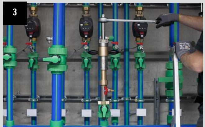
3. Start of the drilling process
