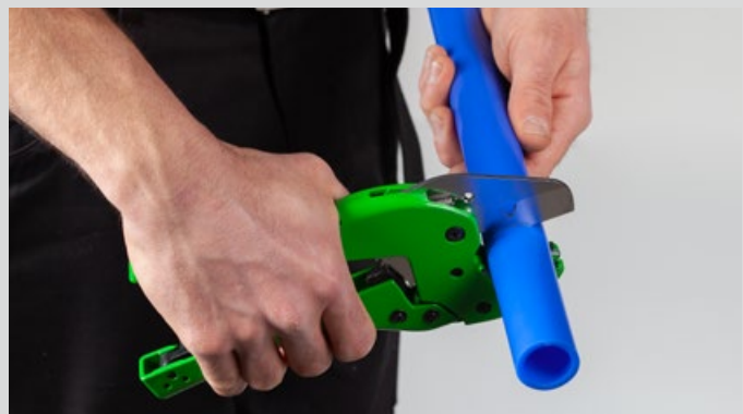
Cutting of the pipe
