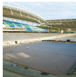
Undersoil pitch heating
